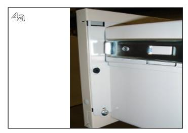
Reinstall the drawers, checking for alignment and fit. Proper spacing at top and bottom is 0.125".
